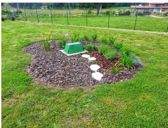
Micro-station Tricel Novo FR6/4000 installée
